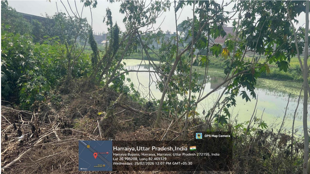
Figure 10: Another Sewage collection pond at Harraiya, UP
